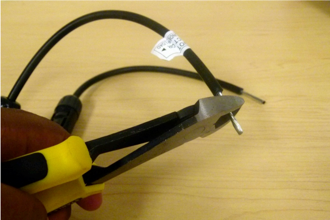
Fig. 3.1. Cutting stripped the end of the 9" MC4 cables to 3/8"
